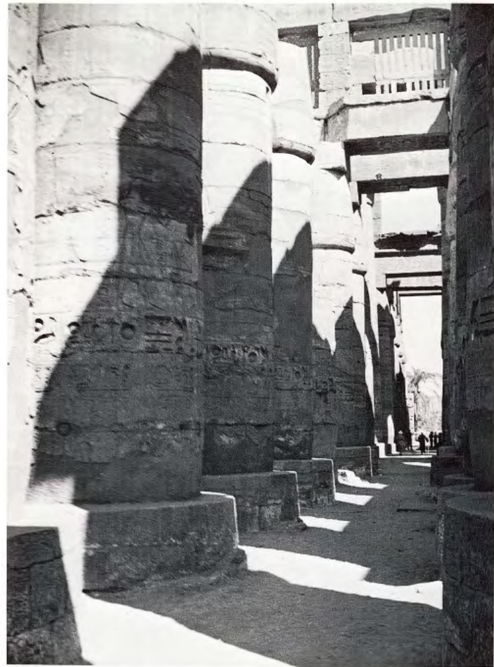
Plate 27. View from the aisle of the hypostyle hall at Karnak (Great Temple of Amun-Re'), showing the clerestory windows bordering the upper part of the nave.
